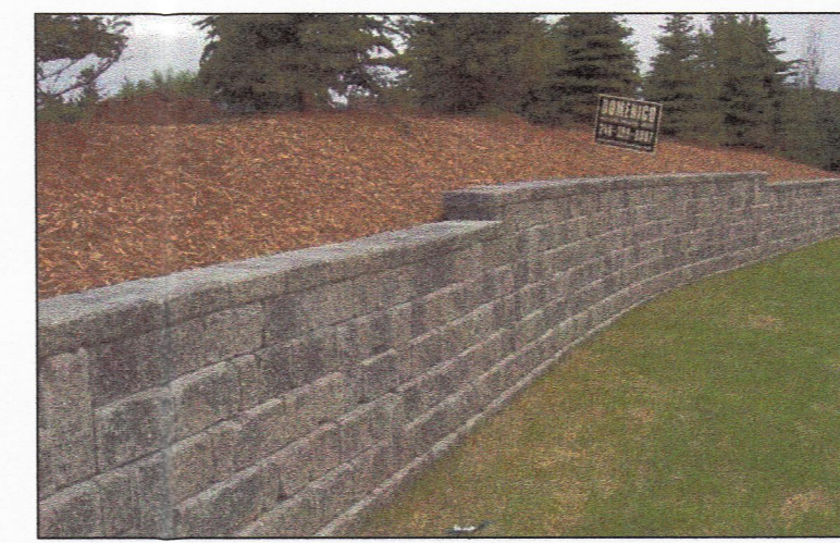
Brick retaining wall
