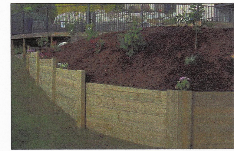
Timber retaining wall
