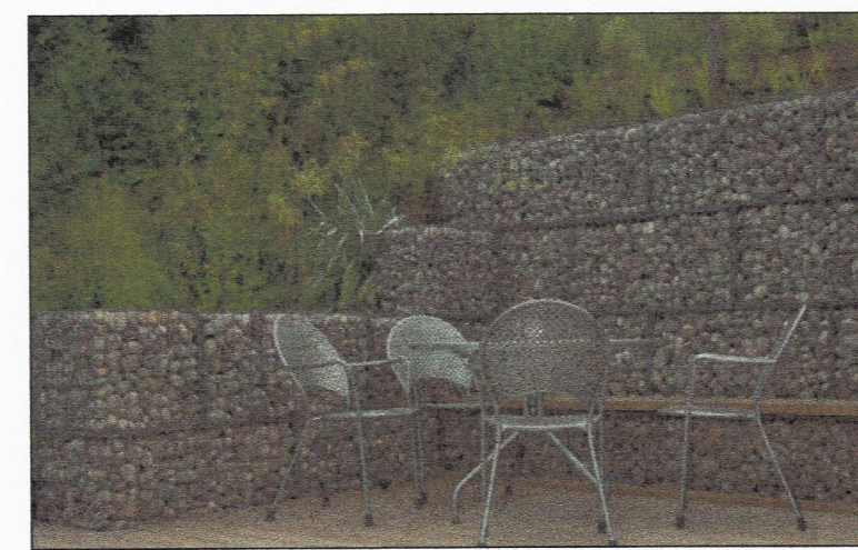
Stone filled gabions
