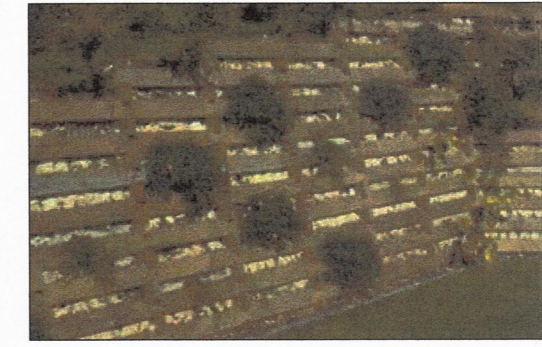
Timber crib wall (with or without planting)
